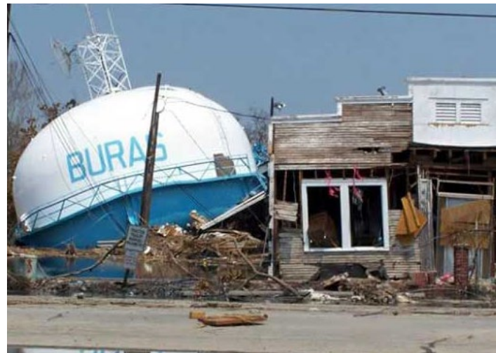
A fallen water tower in Buras-Triumph, Louisiana, where Katrina made landfall. (Source: Wikipedia)
