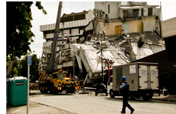
Pyne Gould building destroyed by the 2011 earthquake, Christchurch, NZ. (Source: Wikipedia)
